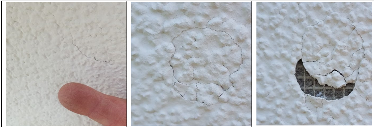
Figure 1. Representations of the damage classes: crack (left), full circle fracture (center) and breakout (right).
