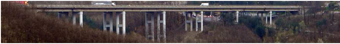
Fig. 3. Lateral view of the Rio Torto viaduct.
